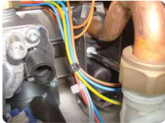
Figure 154 Removal of flat plate heat exchanger (screw on right side) (Combi Only 80/120 shown)
