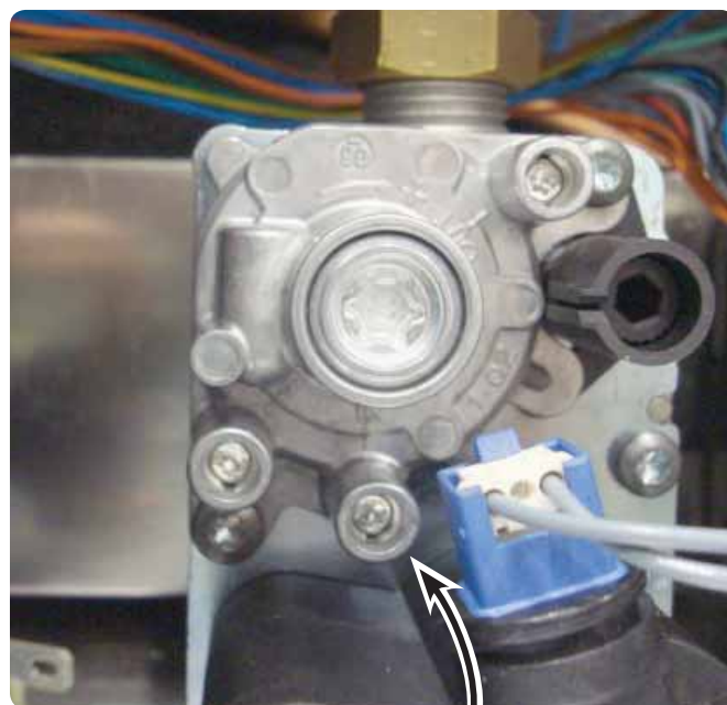
Figure 60 Inlet test port on gas valve
