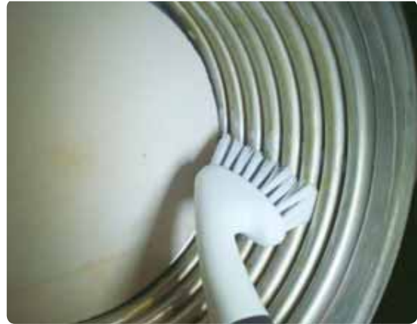
Figure 147 Cleaning the heat exchanger
