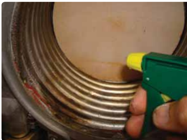
Figure 146 Cleaning the heat exchanger
