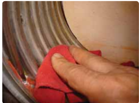
Figure 148 Cleaning the heat exchanger
